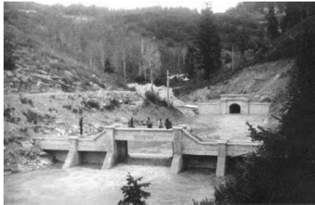
Photograph 5. Water first flowed out of the Strawberry Tunnel, West Portal, on September 13, 1913. Circa 1913.
