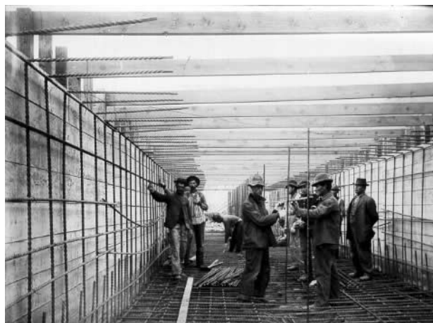
Photograph 12. Construction on a box-flume portion of the Highline Canal Circa 1915.
