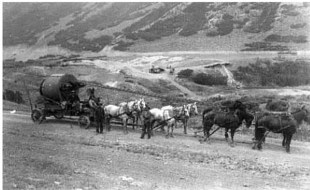
Photograph 4. The majority of the Power Canal traversed steep slopes and had to be concrete lined. Circa 1907.
