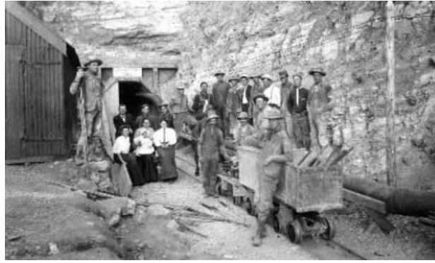
Photograph 1. Force-account crew standing in front of the West Portal, Strawberry Tunnel. Circa 1907
