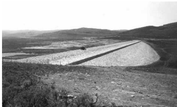
Photograph 10. Hand-laid masonry on the upstream side of the completed Indian Creek Dike. Circa 1912.
