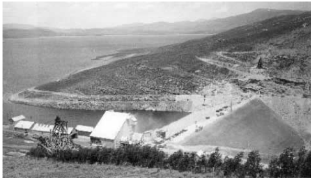
Photograph 8. Crushing and mixing plants from Reclamation Service's Salt River Project, Arizona, were erected at Strawberry during the Summer of 1911. Circa 1911.
